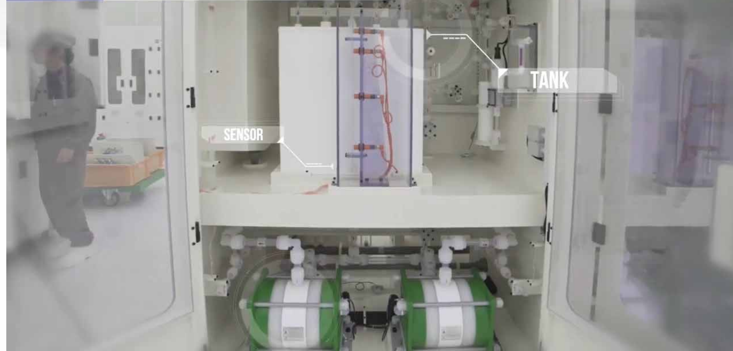
CCSS SYSTEM FOR SUPPLYING HIGHLY PURE CHEMICALS SUCH AS ACID, ALKALI, AND OTHER SOLVENTS
